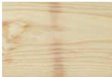
STICKER STAIN: Stain that is typically grey in colour occurring from stickers used to season lumber.
